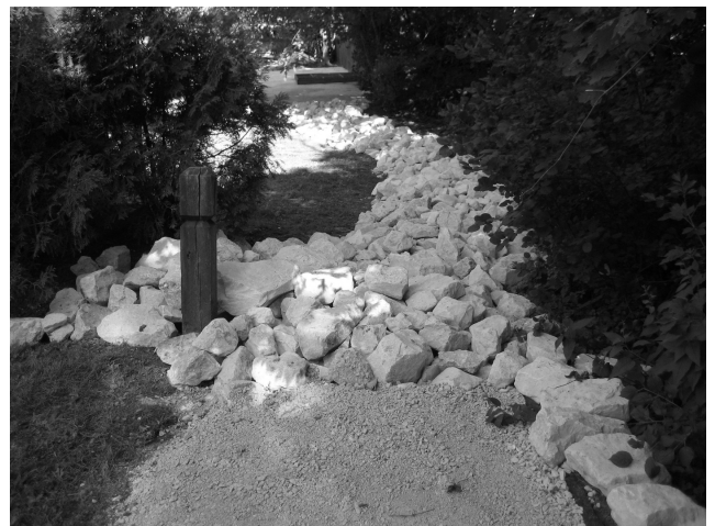
Dry drainage area after improvements.
