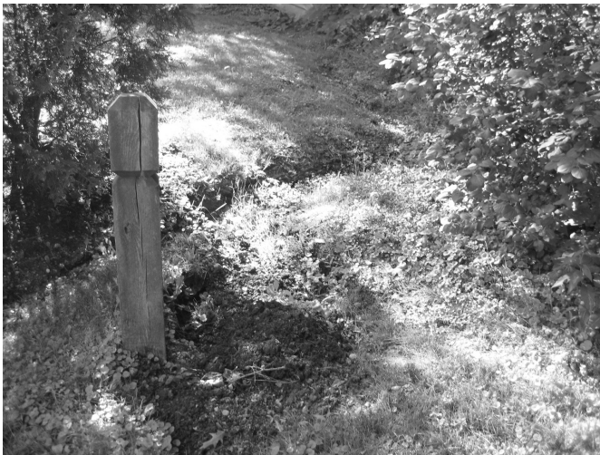
Eroded area in Erker Park before improvements.
